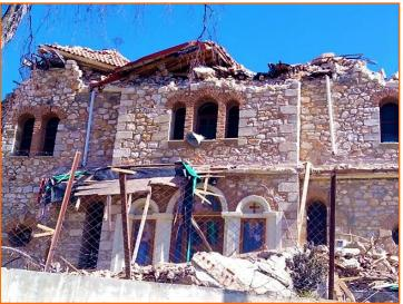
Churches in the earthquake-affected area suffered damage to the load-bearing masonry walls, arches, roofs, plasters and their bell tower.
