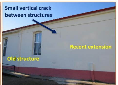
The primary school of Vlachogianni village, where cracks were formed between the old structure and its recent extension due to their different dynamic characteristics. This problem is frequently observed. The solution is simple: either we build the new structure at a distance from the old one, or we adequately tie together the two structures, after a proper structural design.
