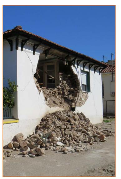
The incurred damage present almost the same manner independently of the mechanical characteristics of the underlying structures. This type of damage (at the center of the perimetric walls), may be attributed to:
