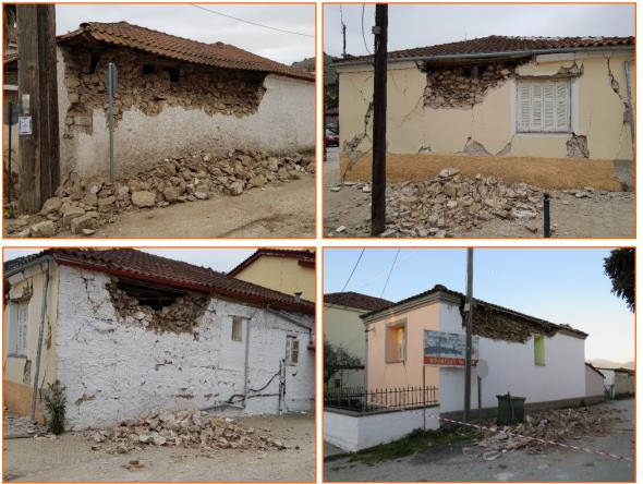
Failures of the upper part of the walls were also attributed to the interaction of roof structure and perimeter walls. This type of damage did not reach collapse condition, but the masonry buildings were unusable during the emergency period. It is also observed that the two layers of the masonry are functioning independently, without connection between them.
