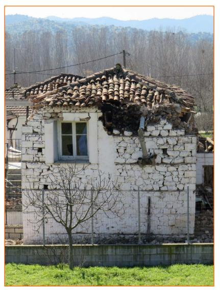
The old unreinforced masonry buildings consist of poor quality mortar. Those types of poor quality mortar are rich in clay, which is highly aquatic. Due to the entry of the moisture into the mass of the wall from the ground and / or from the roof, the friction between mortar and stone blocks, which is beneficial for the strength and stability of the wall, is dramatically reduced until annulated. Actually, the moisture convert clay from a bonding to a slippery material.
