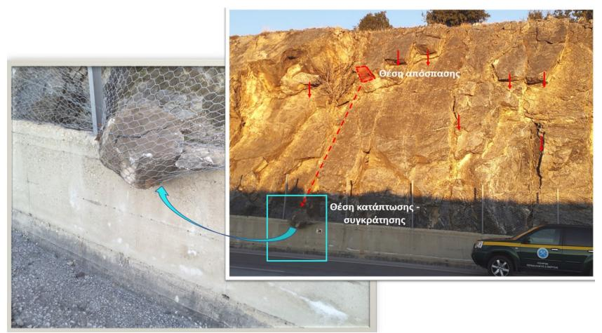
At Meluna, along a slope of the new national road Larissa-Elassona, fragmented marbles fell from heights of 5-30 meters due to the first earthquake. The rock masses that were detached did not cause damage to the road network since the slope failure protection measures worked and the traffic was not disrupted.
