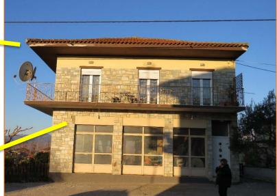
The majority of the reinforced concrete (RC) buildings of the earthquake affected area remained intact by the earthquake. Slight damage was observed to non-structural elements of the buildings. Typical example of slight damage are the detachment and fall of cornices, roof tiles and exterior wall cladding composed of different materials. We observed that the free standing or lightly anchored objects in stiffer structures suffered more damage compared to those standing in more flexible ones.
