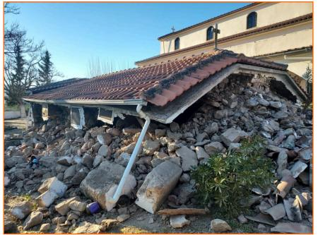
Partial and total collapse of the old and new masonry churches of Agios Nikolaos in Koutsochero village. The old structure completely collapsed, while the new one suffered collapse of its walls behind the altar.
