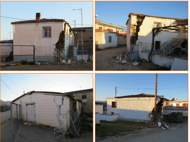
Due to the lack of the aforementioned horizontal band beams, each wall acts individually in in-plane as well as out-of-plane directions under the earthquake loads resulting in vertical cracks at the wall intersections. With these more general views, one could observe the complete lack of diagonal cracks in the masonries.
