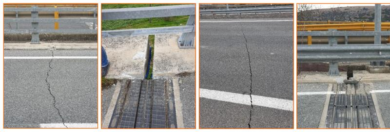
Pounding-induced damages attributed to the presence of these expansion joints were observed in several bridges in the earthquake-affected area. Pineios bridge close to Koutsochero Village is one of these examples.
