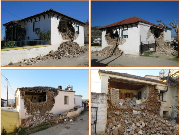
One may well observe the similarity of the incurred damage (at the central part of the walls) independently of the type and the age of the structure. This similarity is due to the same structural scheme and flexibility of almost all roofs. This flexibility is along their vertical axis and is proportional to the ratio of the opening of the roof over the crest height. This ratio is quite large, and it is rather sensitive to vertical vibrations.
