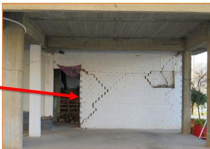
▲ Non-structural damage to building with RC frame and infill walls. It comprised detachment of plaster from the infill walls and extensive cracking of brick walls. The upper floor remained intact by the earthquake. The much softer ground floor is functioning as a kind of base isolator, absorbing thus, in its body, the seismic motion. The observed damage of the few partition brick walls is a physical consequence.
