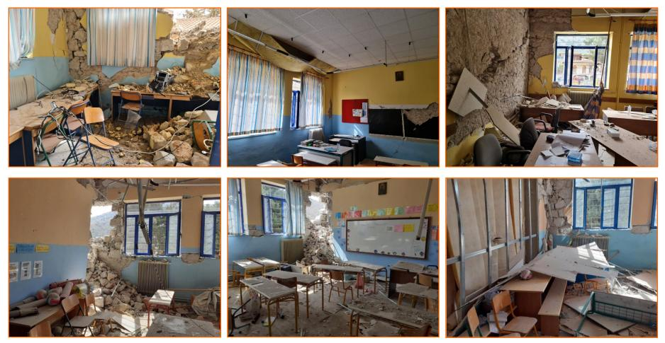
Views of the earthquake-generated building damage from the interior of the elementary school in Damasi village presented in the previous page. The masonry walls partially collapsed affecting only the school equipment.
