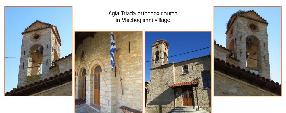
The seismic performance of churches depends on the geological formation of their foundation and on their strengthening. The church in Vlachogianni village remained untouched by the earthquakes. It is founded on alpine formations and moreover it has been reinforced with the installation of steel ties in the bell tower and in the other parts of the construction. The steel ties are placed in critical key points for the stability of the structure.
