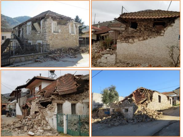
Heavier damage including collapse attributed to interaction of roof structure and perimeter walls. The observed damage are almost symmetrical distributed around the plan of the structure, as shown for example in the top left image.
