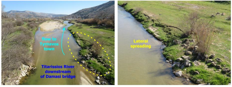
Lateral spreading along the banks of Titarissios River. The site is located downstream of the Damasi Bridge. It is significant to note that the Damasi bridge suffered heavy damage by the first earthquake. Thus, the authorities decided to temporarily close it for vehicles.
