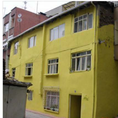
2 nd generation buildings (1970s)
