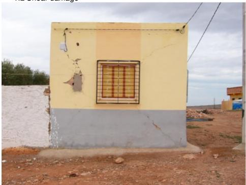
X shear crack in Douria. Grade 2 vulnerability B
