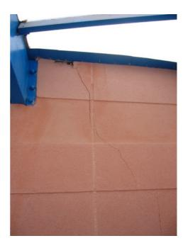
Very slight shear damage to walls and finishes in Nador Airport. Crack below left is cosmetic pounding damage to one side of an expansion joint. Grade 1 or 2 vulnerability D.
