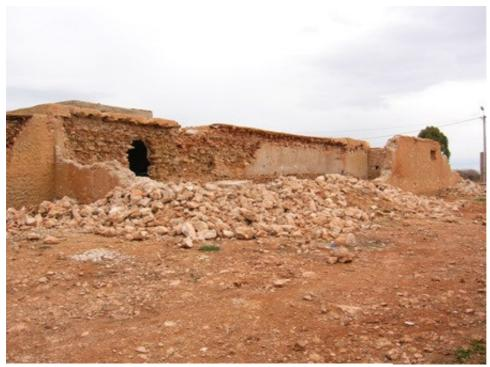
Loss of the outer leaf of a wall and failure of freestanding stone wall in Douria. Grade 3 vulnerability A
