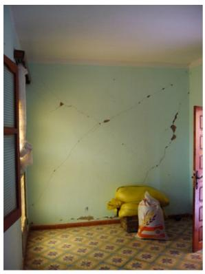
Inside view of crack shown above. Grade 2 vulnerability B
