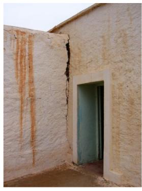
Moderate loss of connection in bearing walls. Grade 3 vulnerability A
