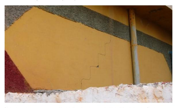
Slight shear damage to concrete block infill wall and parapet in this building in Douria. Grade 2 vulnerability C
