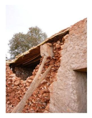
Four views of a damaged composite farm structure with a large concrete beam simply supported on fieldstone bearing walls. Motion of the beam punched the wall out. Grade 3 vulnerability A
