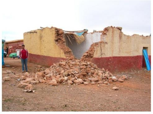
Failed corner and serious damage to roof and walls. Grade 4 vulnerability A
