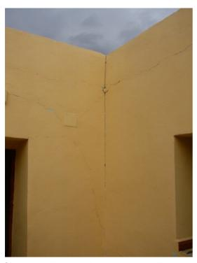
Slight loss of connection in bearing walls. Grade 2 vulnerability B
