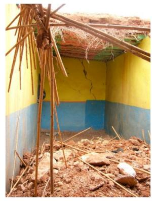
Crack shown above seen from another room with a collapsed previously weakened roof. Final diagnosis is grade 3 vulnerabilidy A
