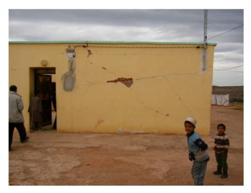
${\sf X}$  shear crack in Douria. Note the vulnerability caused by the existing conduit in the wall. Grade 2 vulnerability  ${\sf B}$
