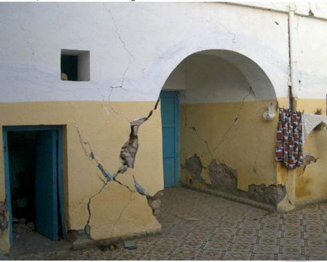
**3.4.3** Shear damage in two perpendicular walls in a house in Tazaghine (grade 3 vulnerability A)
