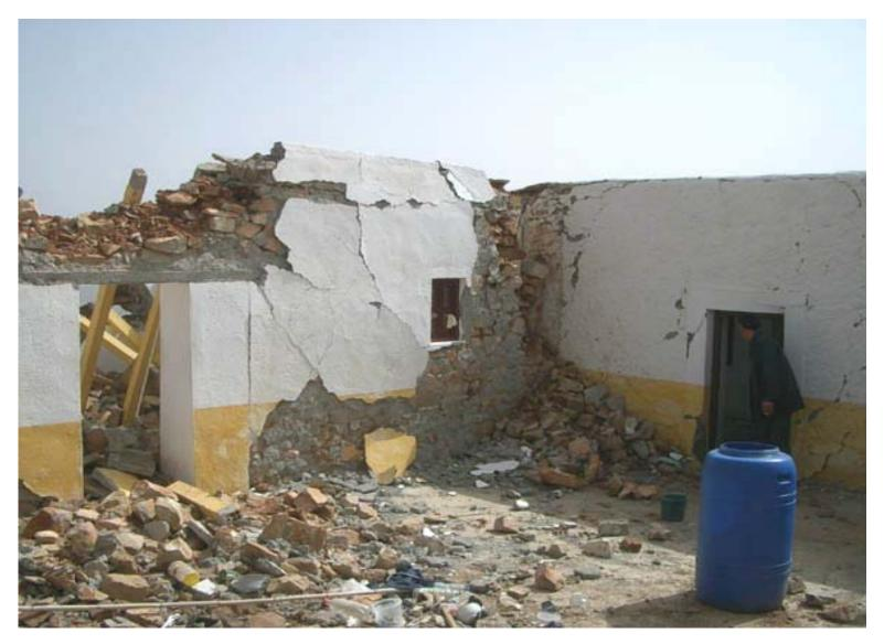
Shear damage to walls and hammering between two perpendicular planes in the corner. 3.11.1
