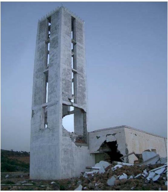
**9.7.1** Pounding damage from the prayer hall to this minarette which is hinging at its 'first floor' level. (grade 3 vulnerability C)
