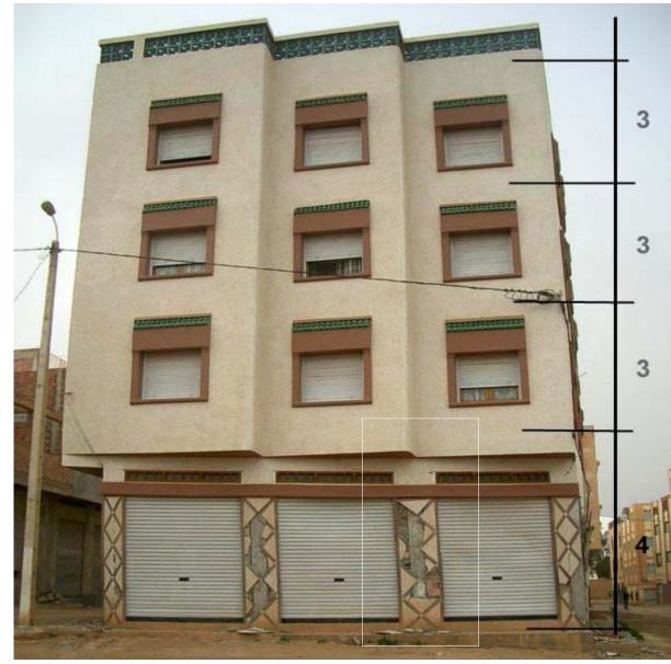
**4.9.1** Open plan shops on ground floor with densly compartmented housing above. This was a classic candidate for soft storey damage. In this building in Imzuren the upper floors have drifted over the ground floor causing plastic hinges and permanent deformations. (grade 4 vulnerability C)
