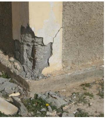
9.6.3 Spalling of concrete; the beginning of a plastic hinge.
