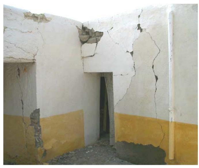
**3.11.2** Shear damage to walls and further hammering damage to the corner.
