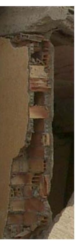
**4.2.3** Close-up of the cavity infill wall.
