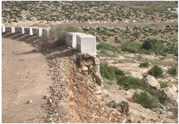
**10.1.3** Collapsed road embankment- Izemurenne
