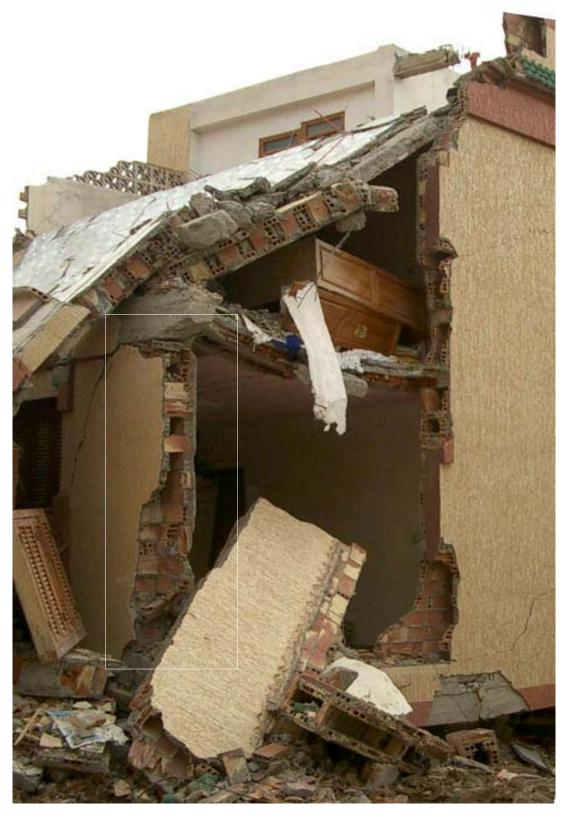
Most RC buildings in Al-Hoceima are clad with a cavity 4.2.1 masonry wall system based on two identical skins of hollow brick external skin construction. units tied together with soldier courses laid across the cavity.
