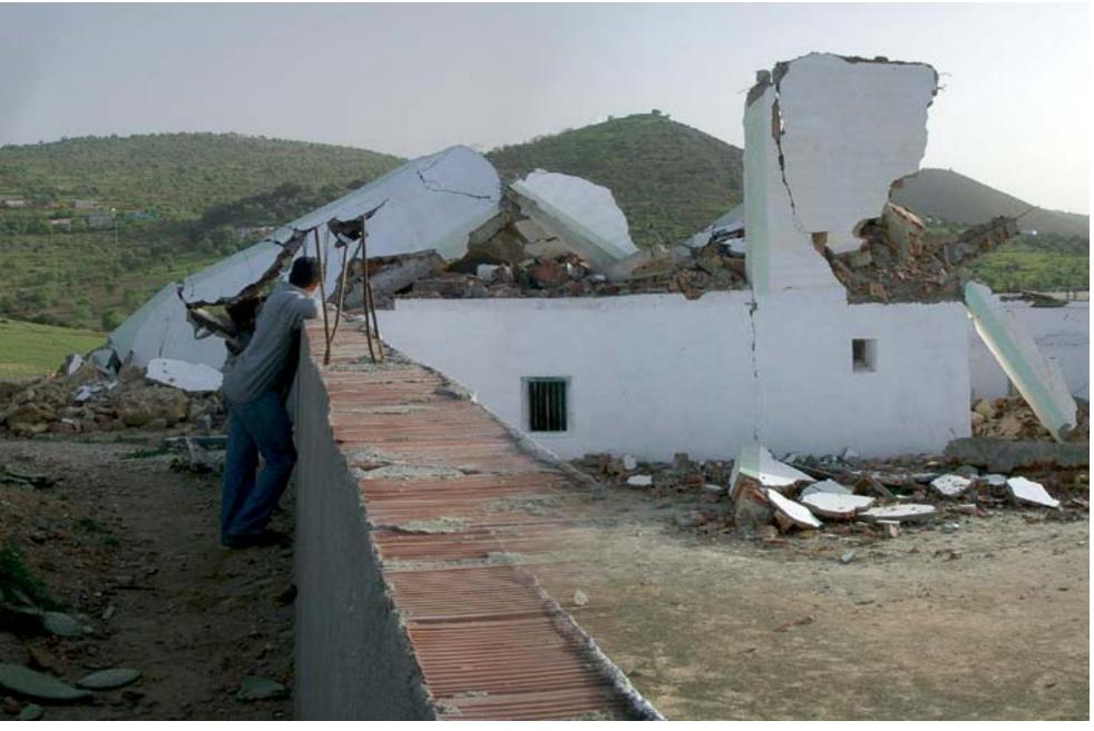
9.9.2 In this case the insertion of the prayer hall building at the base of the tower has caused plastic hinges to develop at the 'first floor' level, as in example 9.7 instead of the ground floor. Toppling therefore, has happened over the prayer hall level.
