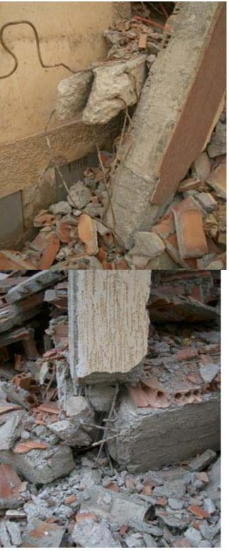
4.1.3 Note the use of non-corrugated steel and inadequate reinforcing layout as well as very small column and beam sections in this failed RC frame building in Imzuren.
