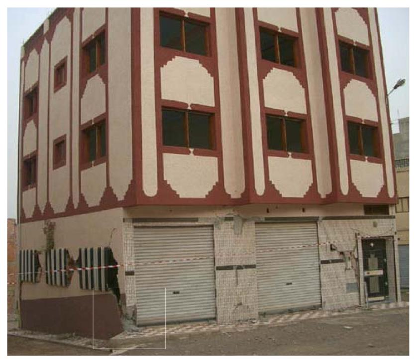
Soft storey damage in Imzuren. (grade 3 vulnerability C) Note plastic hinge on base 4.12.1 of column on a building which appears undamaged at first glance.
