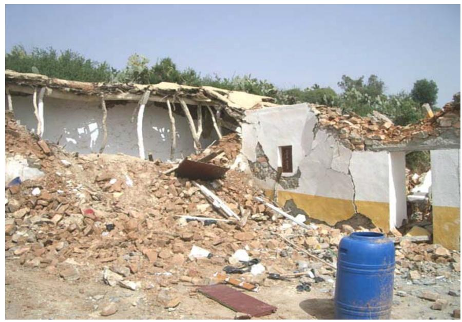
Failure of a loadbearing wall, note the very traditional roofing structure with the wooden posts offering a very 3.12.1 limited diaphragm action. Compare with the better performance in photo 3.12.2
