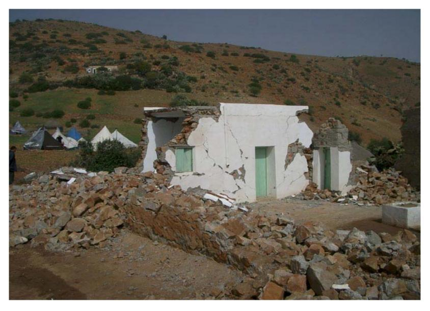
**3.6.2** Same building from a different angle, incorporating failure of freestanding patio masonry wall. Refugee camp in the backround.
