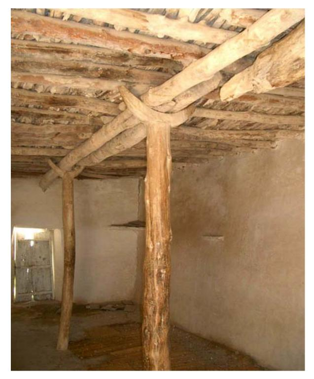
2.2.2 Traditional roof construction incorporating wooden posts. There is very poor diaphragm action in this type of construction.
