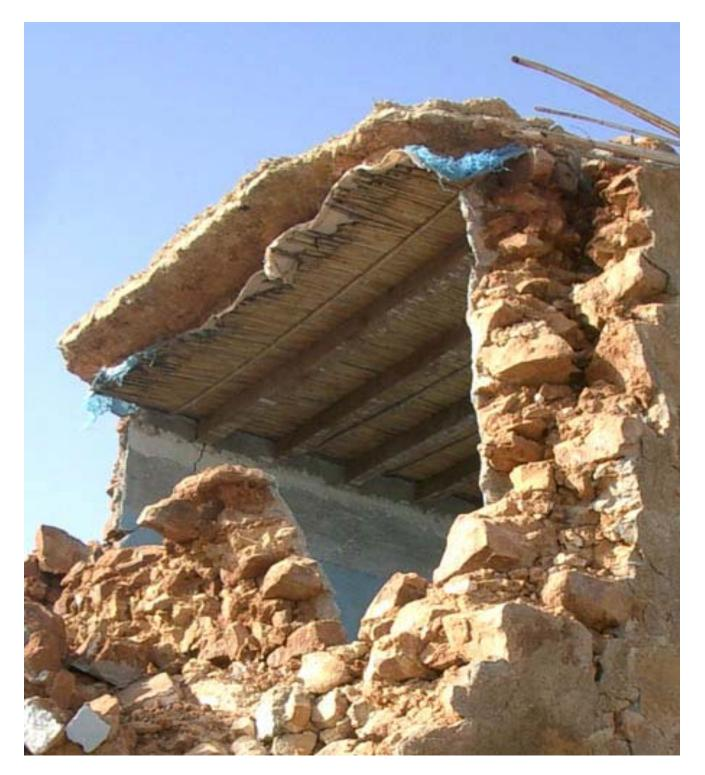
Traditional roof construction with a mortar screed laid over canes and wooden 2.2.1 joists, a weak diaphragm action.
