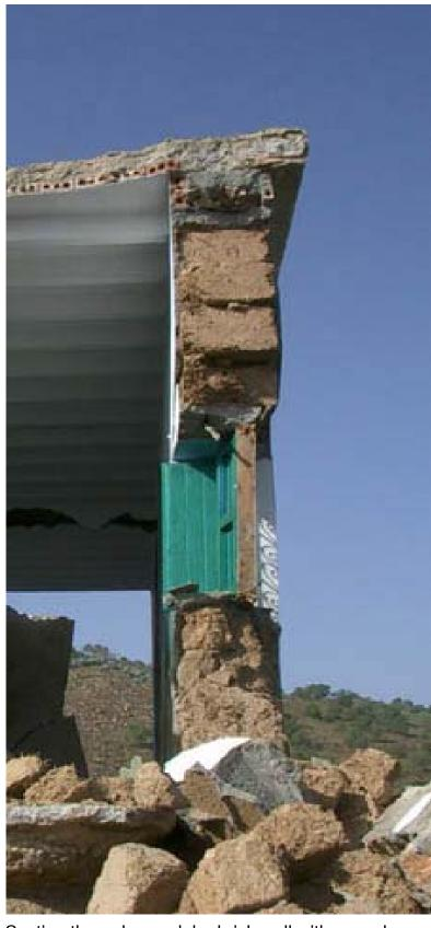
2.1.1 Section through a masonry wall with fieldstone arranged in a weak mortar. The bond is irregular but the stones are sorted to form an internal and external face. With time, the weaker fill material deteriorates resulting in two independent walls.
