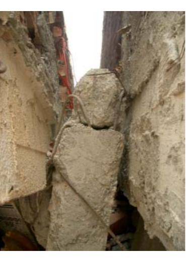
7.2.3 Column head detail. Note plastified noncorrugeted steel and small column section.
