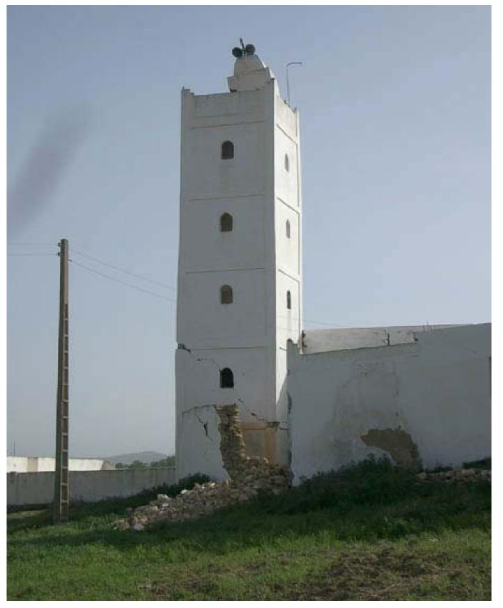
9.4.1 Lantern collapse and shear damage to base of tower. Note simple toppling failure of closure wall. (grade 3 mixed vulnerability A+C)
