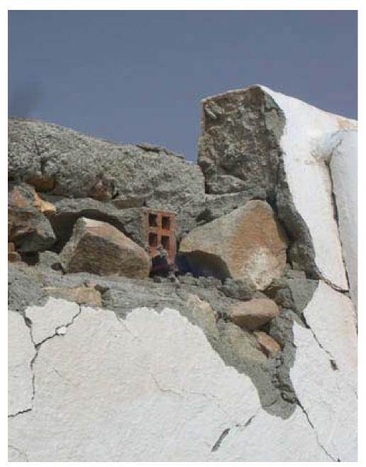
2.3.1 In today's traditional construction, small beams are cast using bricks as formwork, incorporating a single rebar for small spans in housing. Although hardly a moment resisant connection, there are shades of increased performance by the semi-diaphragm action resulting from this construction detail.
