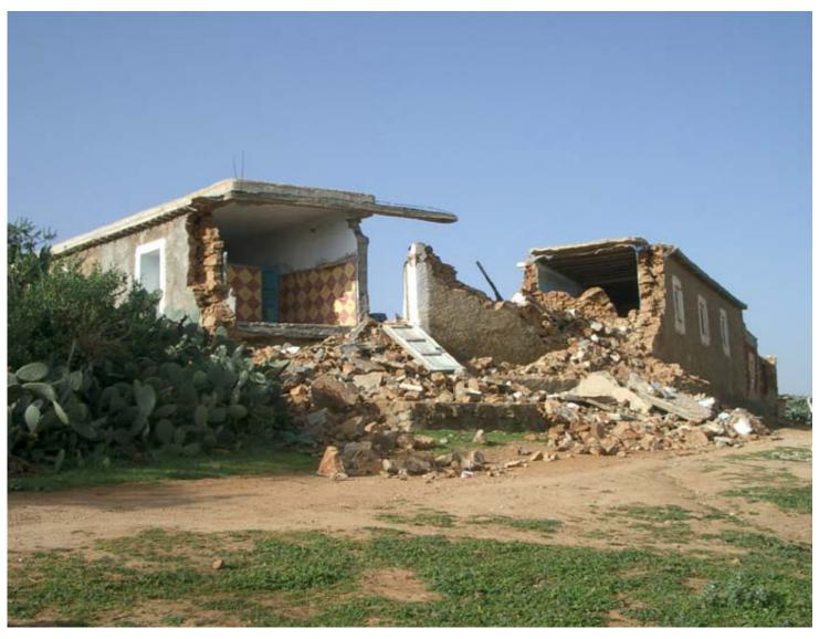
3.7.2 Advanced corner failure and loss of unsupported gable wall. Aït Jamra. (grade 4 vulnerability A)
