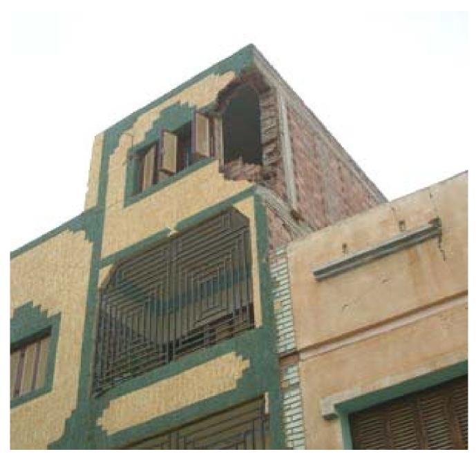
4.4.1 This loadbearing wall has failed in a characteristic corner failure as observed in loadbearing masonry construction, resulting from being horizontally loaded by a very unstiff RC frame in this building in Imzuren. (grade 2 vulnerability C)
