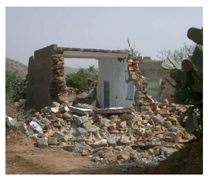
Corner failure and loss of unloaded gable wall. Ait Jamra (grade 4 vulnerability A) 3.6.1
