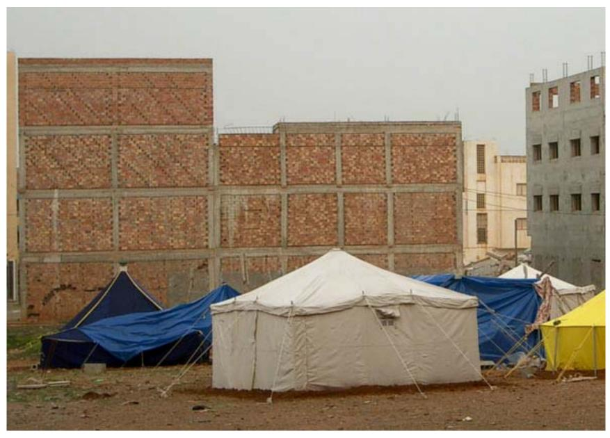
4.3.1 The lack of stiffness of the main RC structure is compensated by the participation of the hollow brick infill panels, which provide an added rigidity to the whole, in particular in those floors densly divided into flats. The unforeseen participation of the brick partitions single them out as especially vulnerable to damage and as we shall see later, can modify the response of the structure. (grade 2 vulnerability C)
