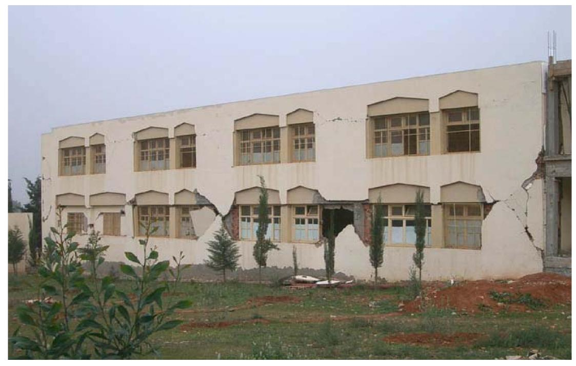
4.6.1 Extensive shear damage to non-loadbearing external walls in this RC school in Imzuren. (grade 3 vulnerability C)
