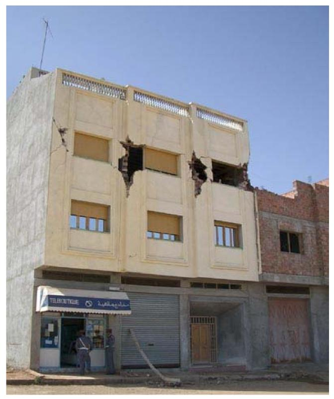
**4.7.1** Pounding from the shorter stiffer building on the right has caused localised damage at the level of impact in this building in Imzuren. (grade 3 vulnerability C)
