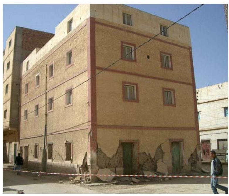
3.4.1 Shear damage to the piers on the ground floor of this unreinforced brick and stone masonry building in Imzurén. (grade 3 vulnerability A)
