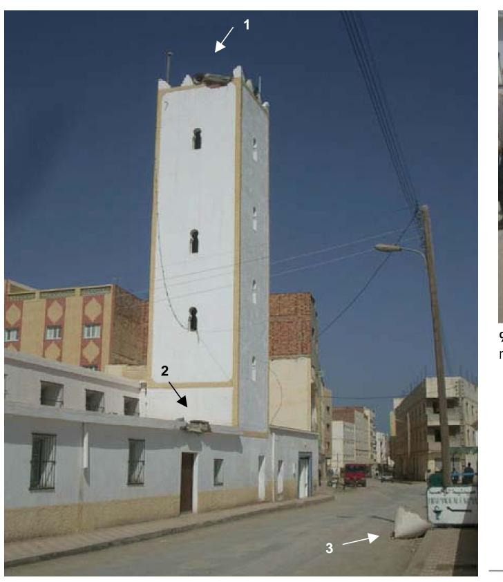
9.5.1 Here the lantern was knocked over (1) striking the entrance area (2) finally rolling over the road. (3) (grade 2 Vulnerability C – some may argue grade 3 'chimneys break at roof level') **9.5.2** Remains of the cupola on the road.
