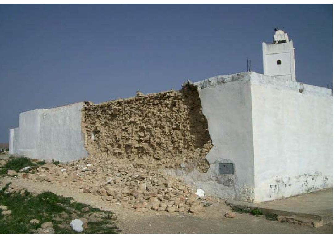
Loss of the external wall of this masonry loadbearing wall in a mosque in Izemurenne (grade 3 vulnerability A) 3.2.1
