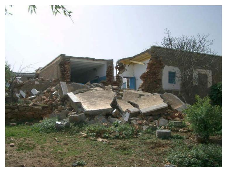
Advanced corner failure with loss of roof slab. Aït jamra. (grade 4 vulnerability A) 3.7.1
