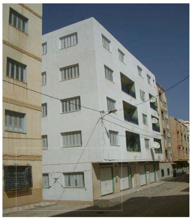
**4.5.1** This non structural partition wall has been damaged by shear after being loaded by the movement of the RC structure of the building. Imzuren. (grade 2 Vulnerability C)
