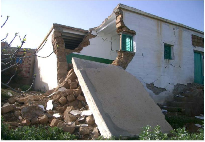
Advanced corner failure can cause the roof slab to collapse. (grade 4 vulnerability A) 3.5.3
