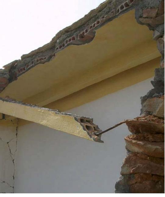
**2.3.3** View of a failed 'beam' as detailed alongside.
