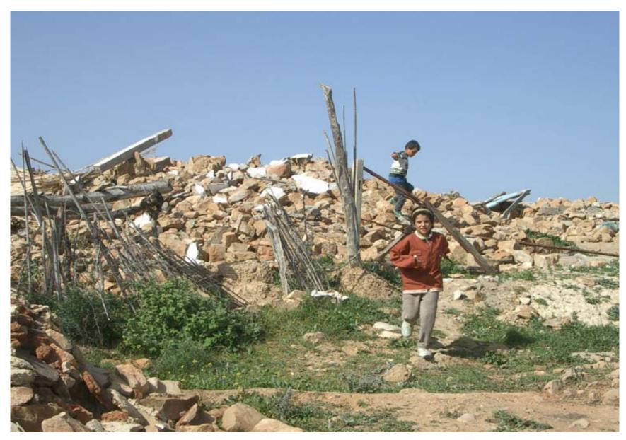
In the chaotic damage of grade 5 it is often difficult to discern the original form and plan of the building, 3.8.1 and is thus of limited use for damage analysis.
