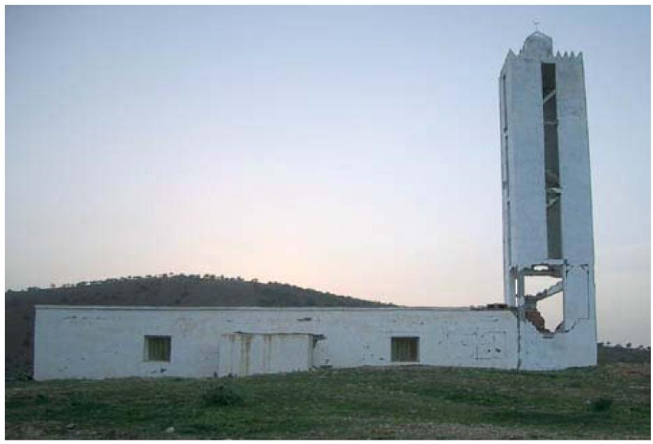
**9.7.2** side view. Note the low long and stiff prayer hall's pounding damage to the diaphanous tower.
