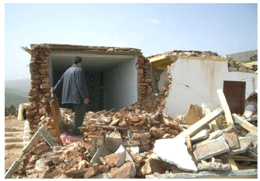
Corner failure and loss of the end gable wall has caused the collapse of the dormory wing of this 3.10.1 house and killed the wife of the owner. He is standing on the remains of the bed. Note the exposed wall construction and how it has been cracked into two skins.
