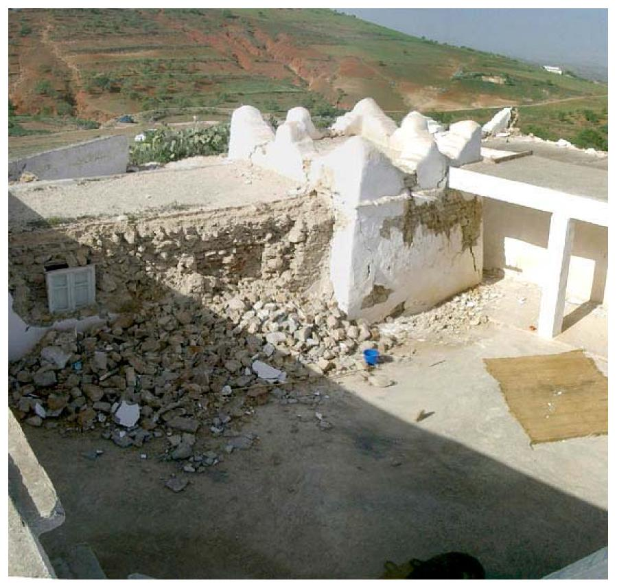
**3.3.3** Failure of external skin in this masonry wall in a mosque in Ait Jamra. Note that the loss of a whole skin has not jeopardised the load bearing ability of the whole. (grade 3 vulnerability A)
